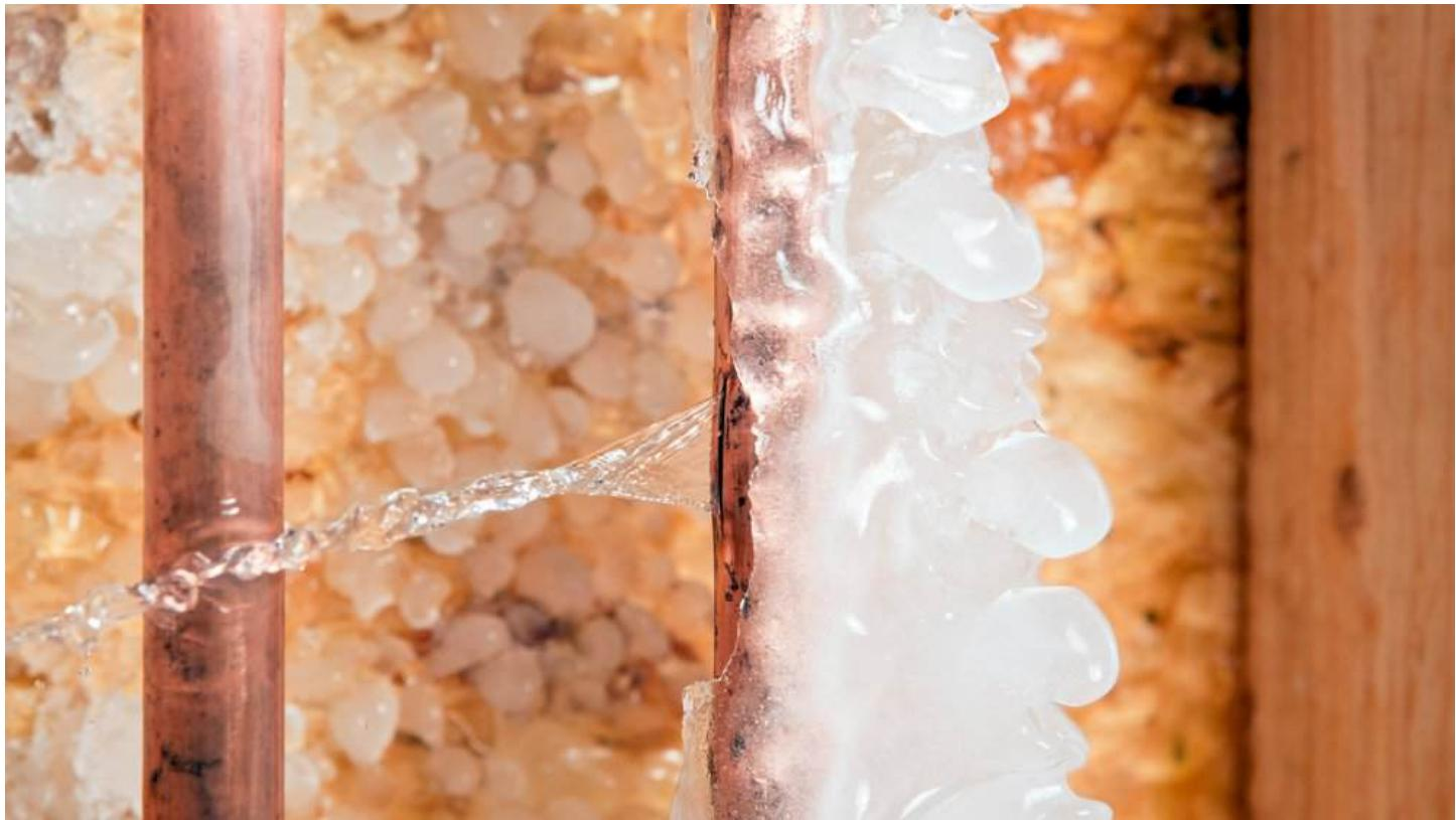
It's that time of year again: cold snap season. Plumbing systems can freeze when temperatures take a sudden nosedive past the freezing mark, or 32 F. And when water freezes and expands within a pipe, the pipe can burst.
